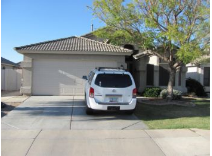
Exterior General condition
